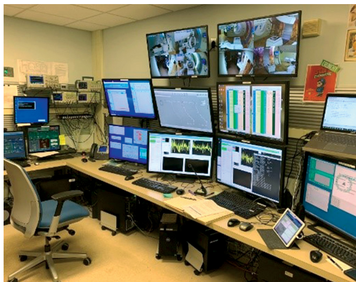
CONTROL ROOM AND BEAM MONITORING
